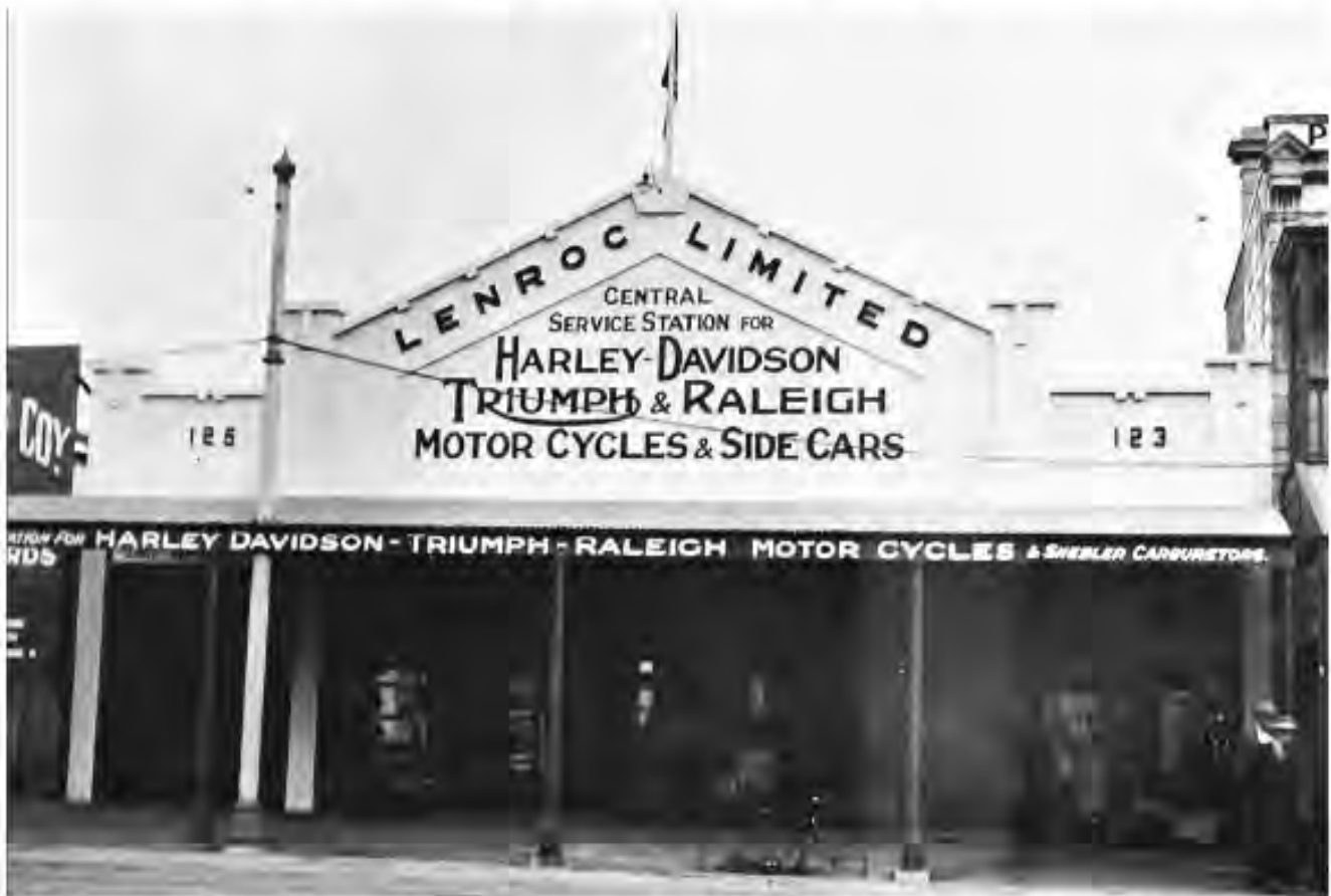
Lenroc's building on the south side of Flinders street in 1924. They later expanded to the west to deal with used cars.
